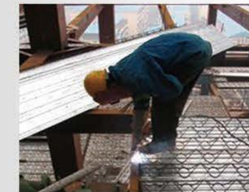
5. 垂直支持鉄筋の電気溶接 Point welding the vertical bracket rebar
