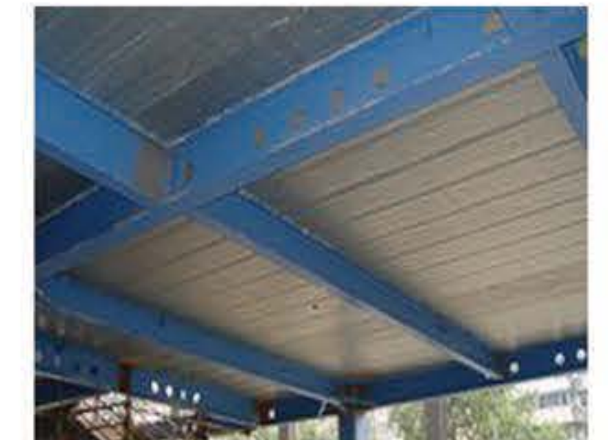
12. 打設完了時の底部効果 Bottom effects after placing concrete
